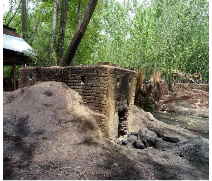
Fig. 14: A damaged boiler
